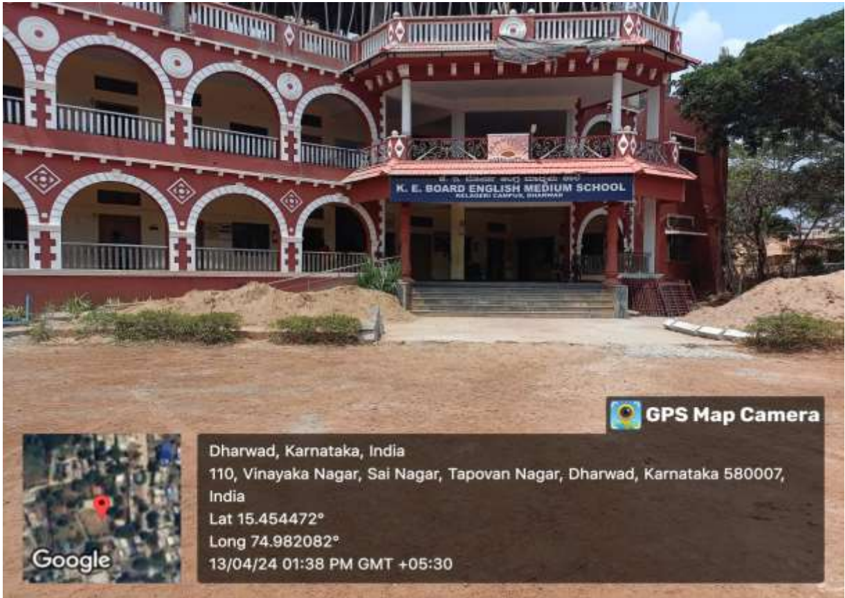
SCHOOL FRONT VIEW
